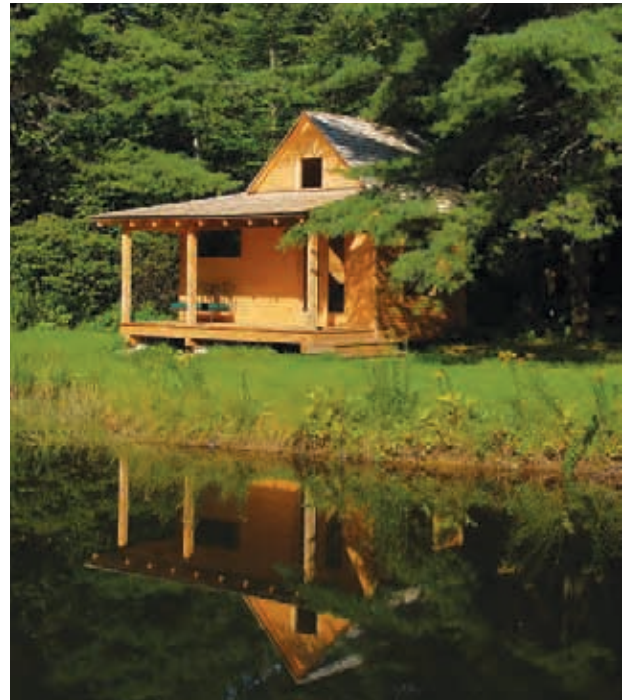
This sauna-cum-teahouse, tucked away on the flanks of the Green Mountains south of Middlebury, is a lovely example of global design, local execution. Elizabeth Herrmann architecture + design took inspiration from the owners' travels in Japan and Finland, and Northern Timbers built the structure of green wood from a local mill; www.eharchitect.com .
