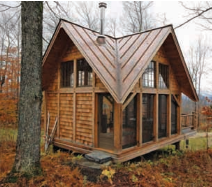
This Waitsfield timberframe teahouse by Birdseye Design makes the most of a beautiful view in a wooded setting. It features cedar panels set within the timberframe, copper standing-seam on a cross-gabled roof, and clerestory glass set within the steep gables; www.birdseyebuilding.com .
