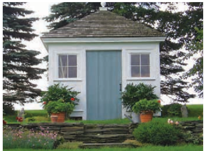
This classical Colonial toolshed in Woodbury, designed by Pat Pritchett, provides functional storage for all the tools and equipment of an avid gardener; www.vermontvernaculardesigns.com .
