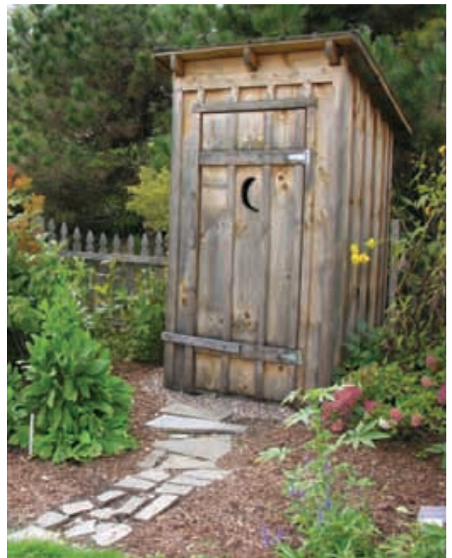
This charming outhouse, designed by Richard Gamache of Swanton, is one of several small garden structures in South Burlington's Vermont Garden Park.
