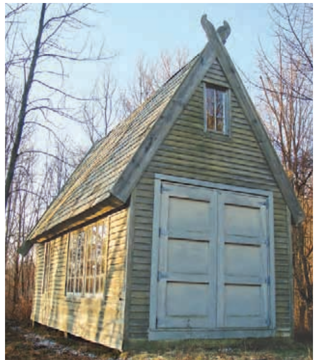
The crossed Viking horn finials atop the roof peaks of this East Dorset structure announce the Scandinavian influence that inspired designer Marta Elise Johansen. The slate-roofed, cedar-sided building contains a studio for art or writing, a sauna, and a sleeping loft; www.martajohansen.com .
