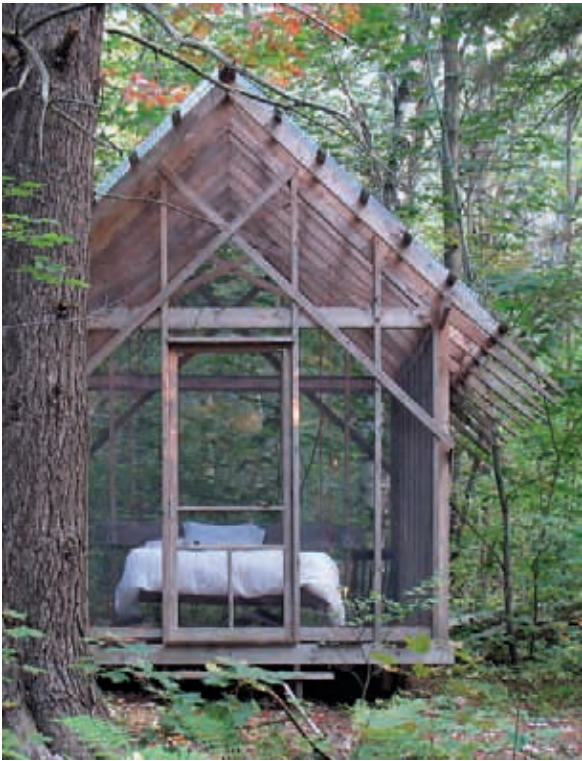
Who says an idyllic retreat needs to be elaborate or expensive? Robert Swinburne of Halifax built a simple 2 x 4 frame, wrapped it in insect screen, and used parachute cord to suspend the bed from the clear polycarbonate roof. His Fern House appears to float atop a sea of ferns; www.swinburnearchitect.com .
