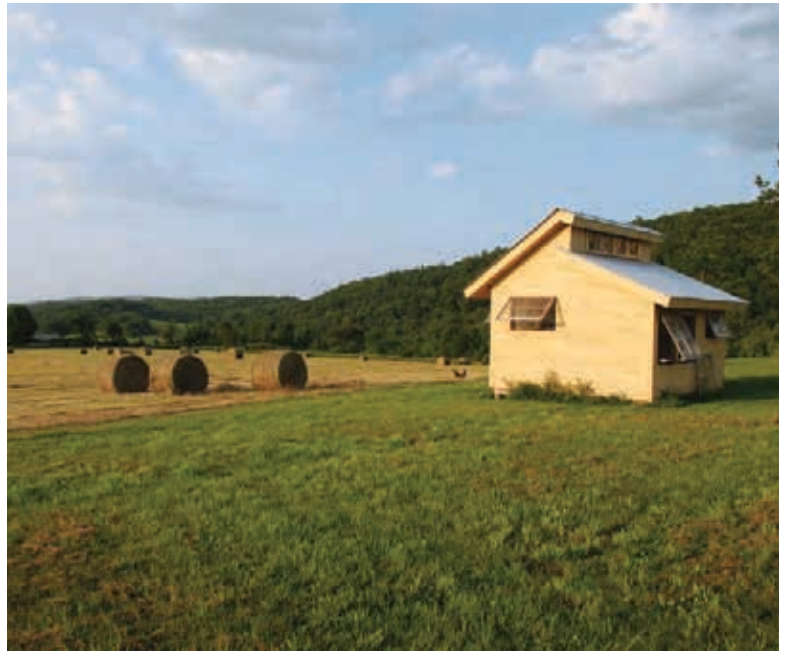
Built primarily of salvaged materials, David Pill's hen house in East Charlotte fits perfectly into a landscape designed in accordance with the principles of permaculture and a low carbon footprint; www.pillmaharam.com .
