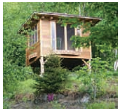
Students in the Yestermorrow Community Design/Build course created this mountaintop teahouse in Roxbury. It was designed by architect Mac Rood; www.yestermorrow.org .
